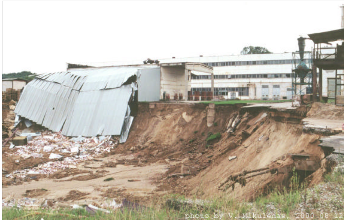
Figure 7.1 Landslide head scarp and destroyed storehouses
