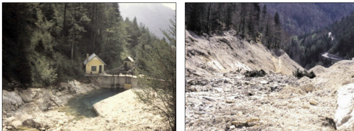
Figure 3.2 Mangart hydropower plant before and after its destruction by the landslide of 15 November 2000 (photograph: archives of the PGD Log pod Mangartom)
