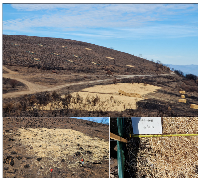
Figure 6 – Experimental and operational mulch treatment implementation in Yeres wildfire (Castilla y León, Spain), Sept. 2025.
